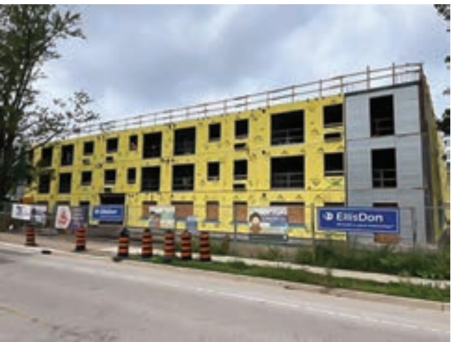
Here are Canam's exterior load-bearing steel studs with yellow, dense glass sheathing. Also, shown on the far right, is the Canam concrete shearwall. pleting the design by April was the real challenge rather than the fabrication or construction phases. "That accelerated design was achieved in about half the time a similar design project of this scope would normally take. We (EllisDon) couldn't have done it without Canam," says Stewart. A fast tracking approval process by the City of London also expedited the project, he points out. Construction continues at 122 Baseline Rd. W. and some of the work still left to be completed by EllisDon's own 60-member workforce includes apartment unit fit outs and the erection of the building envelope which will consist of brick veneer, says Stewart. EllisDon is also working with Housing Development Corporation London on the planning and design of similar affordable housing, he says. Housing Development Corporation London, a non-profit agency whose mission is to provide housing for low income and vulnerable residents, was able to access just over $7.5 million in federal funding to offset the $17.5 million cost of constructing the building on municipal surplus land which the City of London had transferred to the corporation a few years ago.
