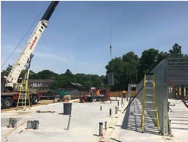
Setting a Canam load-bearing interior corridor wall on to slab on grade at the 122 Base Line Rd. W. project in London, Ont. Slab on grade poured June 23, 2021.
